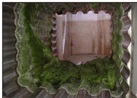
ABOVE: Cleaning systems prevent algae from growing on the UV lamps, but not on the mounting hardware. RIGHT: Algae flourishes on the stainless-steel environment of the UV reactor.
