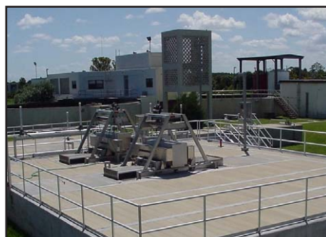
RIGHT: The four banks of UV lights are installed on top of the reactor channel. ABOVE: A view of one of the UV light banks raised out of the water for maintenance.
