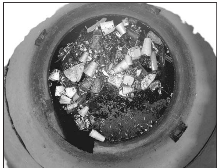
Pollutants trapped in the CDS sump can not be flushed back into the drainage system.
