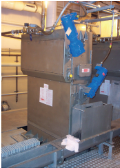
Figure 2. Typical Installation of a Band Screen
