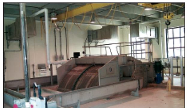
Figure 4. Typical Installation for a Drum Screen
