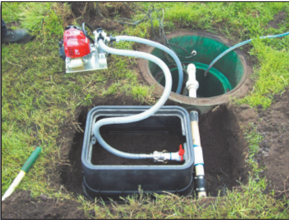
Figure 3. Recent Field Construction Test Model
