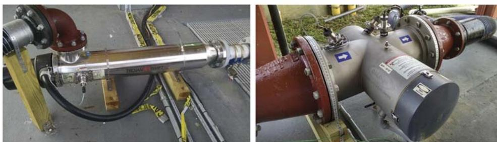
(a) Low-Pressure High-Output and (b) Medium-Pressure
