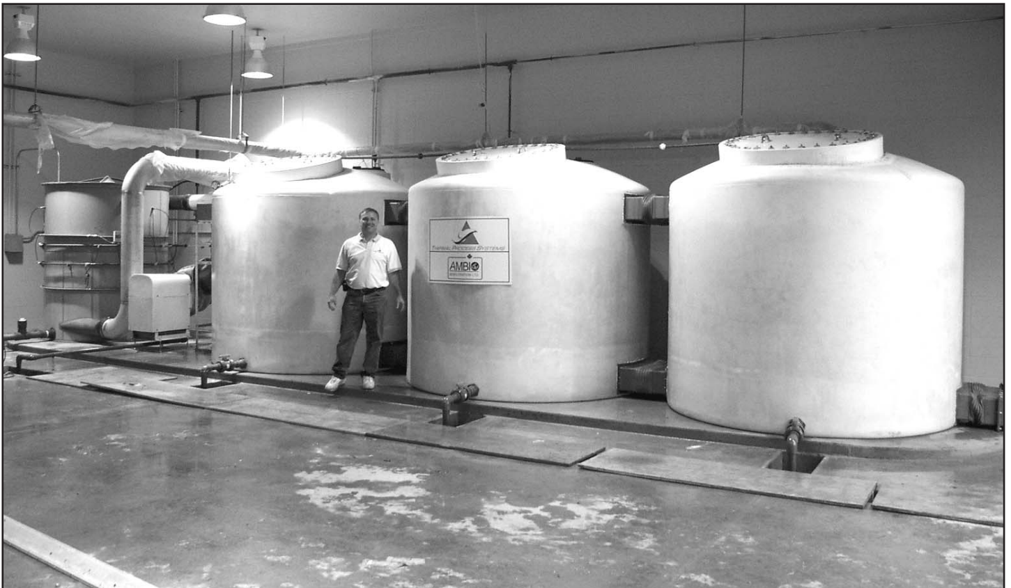
Modular biofilter bed system (top down air flow), treating 600 cfm of ATAD air, Franklin, Indiana
