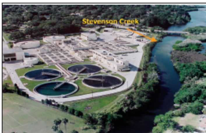
Figure 1 – 10 MGD Marshall Street APCF discharging to Stevenson Creek
