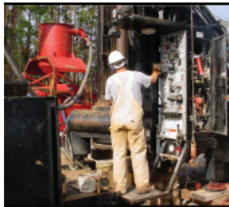
Figure 4: Photograph of the Drilling Equipment
