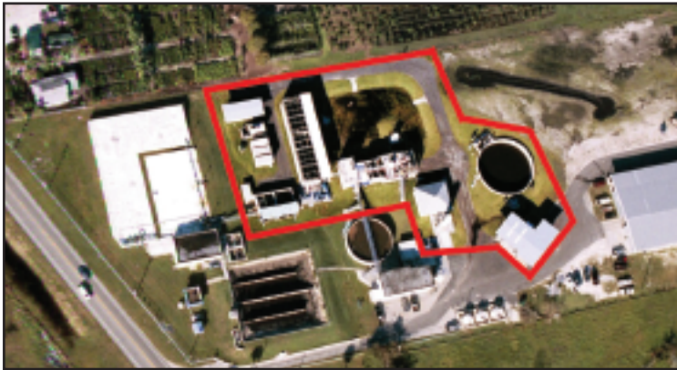
Figure 1: New Water Treatment Plant Facilities
