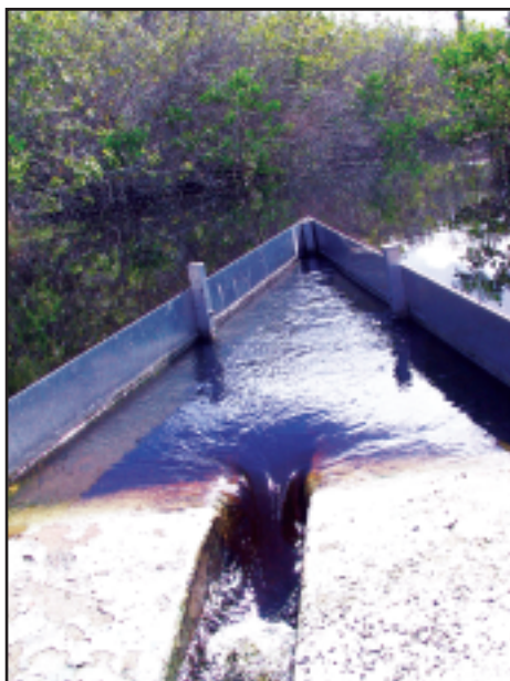
The Outlet Water Control Structure consists of a level-lip weir with a bleed-down notch and a skimmer.
