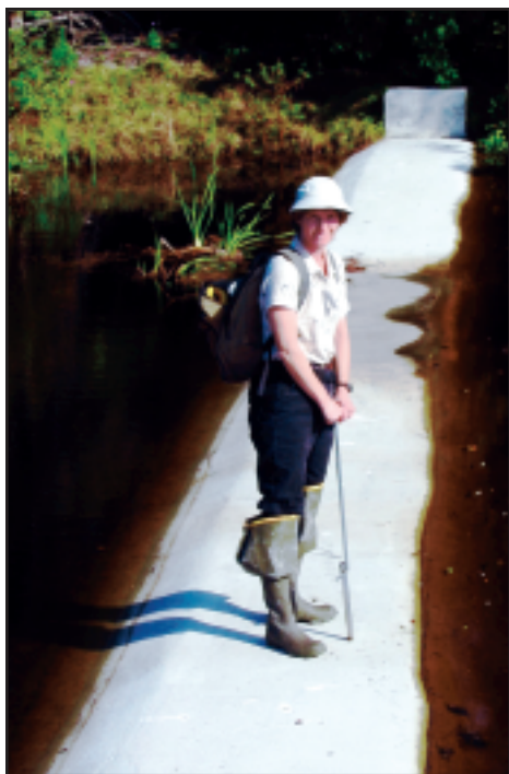
One of the six level-lip spreaders that distribute pretreated stormwater runoff into the VAB Wetland.
