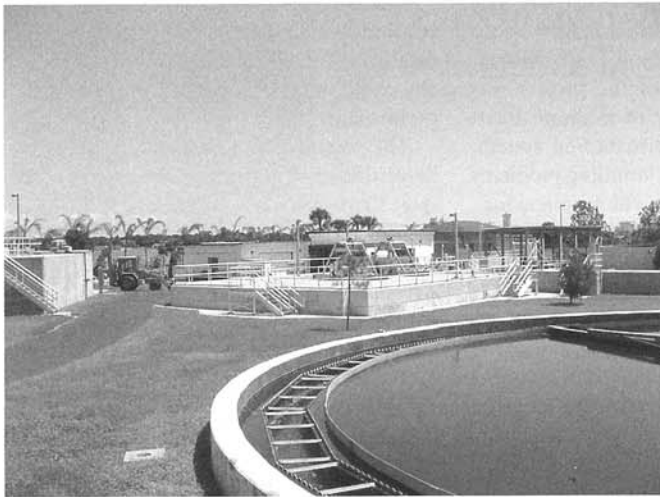
Bethune Point is situated along the west bank of the Halifax River. McKim & Creed increased capacity at the plant from 10 to 13 mgd; converted the treatment to a safer, cleaner UV system; changed the process to a Bardenpho system; and incorporated a UPS system.
