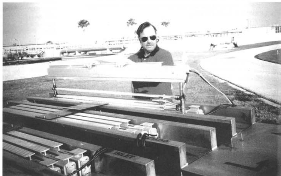
Bill Banks, plant superintendent at Bethune Point, inspects low pressure, low intensity UV lamps.
