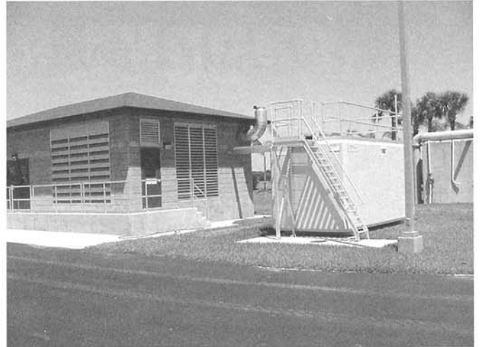
The MDP (Master Distribution Panel) / Generator building and the 6,000 gallon above ground fuel tank at Bethune Point. The structure was designed so the floor slab is above the 100-year flood elevation; hence the two-plus foot difference between floor slab and existing grade.
