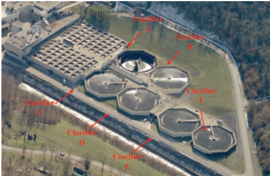
Figure 1. Aerial View of the Kentucky Wastewater Treatment Plant Final Clarifiers
