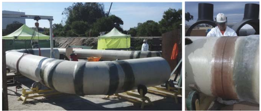
Image 2. Fiberglass Field Laminations
