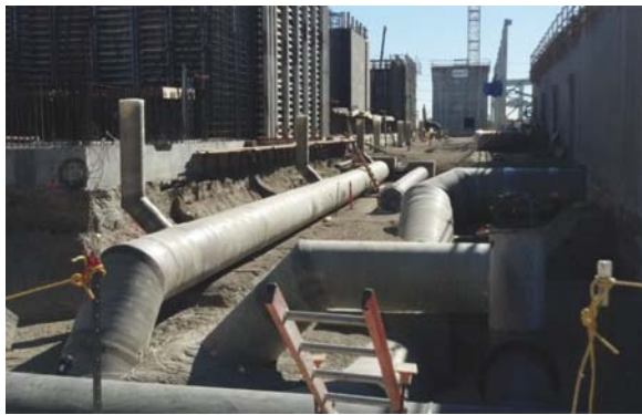
Image 1. Fiberglass Pipe Installation
