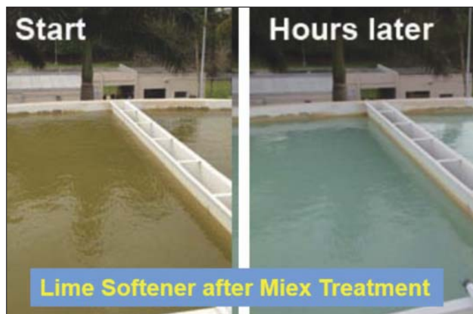
Figure 1. Water Treatment Plant No. 2 Lime Softener
