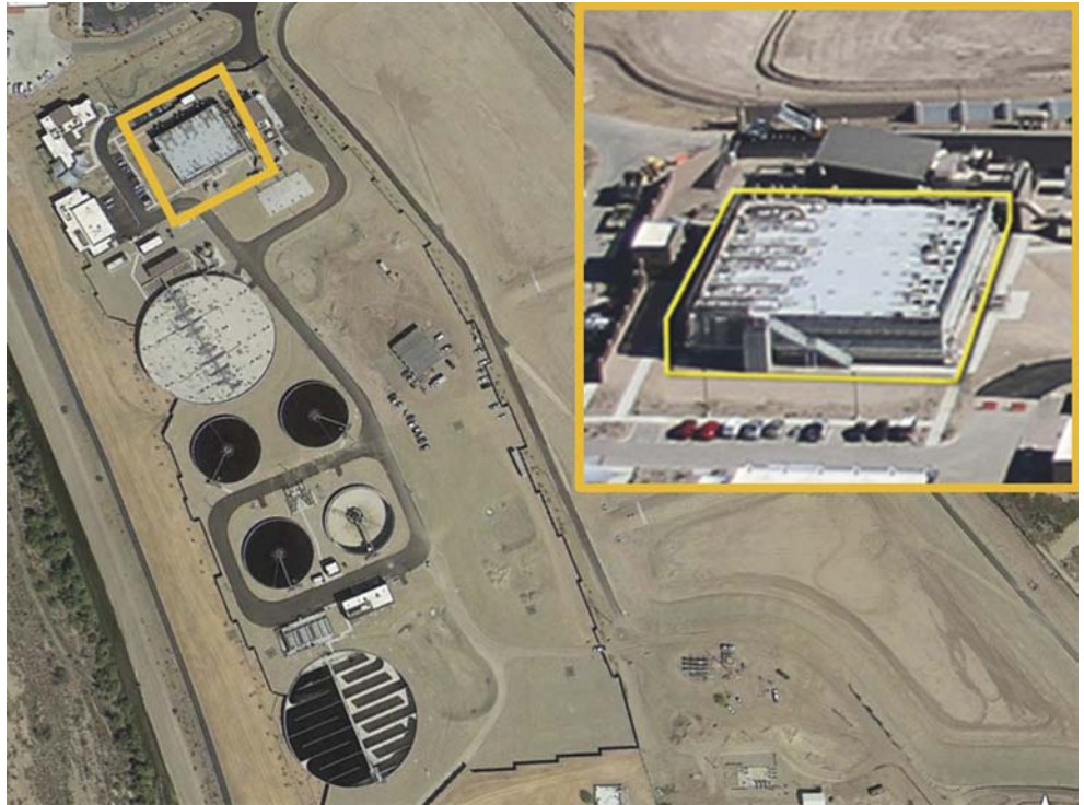
Figure 3. Aerial view of the biologically enhanced primary treatment process at the Agua Nueva Water Reclamation Facility. (photo: Pima County)
