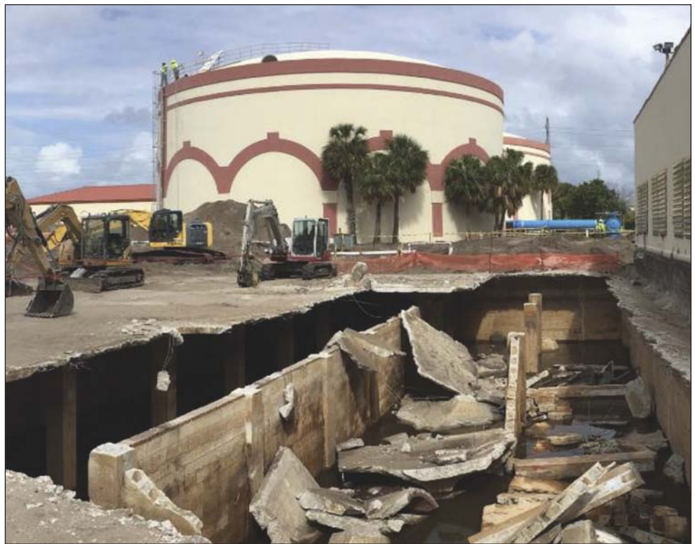
Figure 8. Clearwell Roof Demolition (photo: Stantec)
