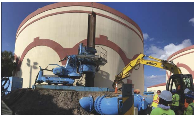
Figure 5. Push-Sheeting Installation Around 3-MG Tank (photo: Stantec)
