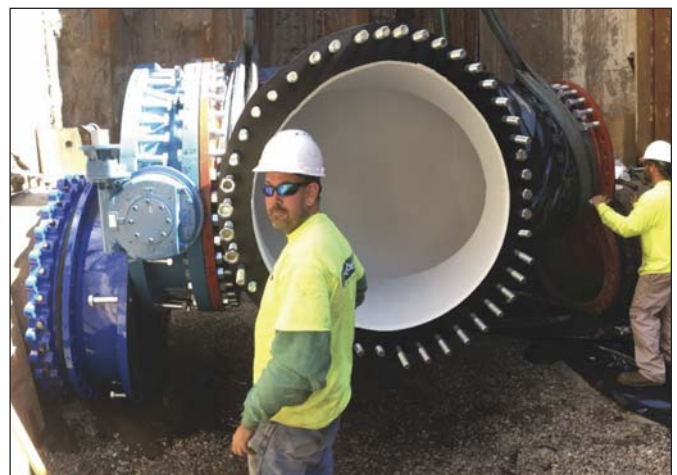
Figure 6. Custom 48-in.-by-36-in. Reducing Tee Fitting Installation
