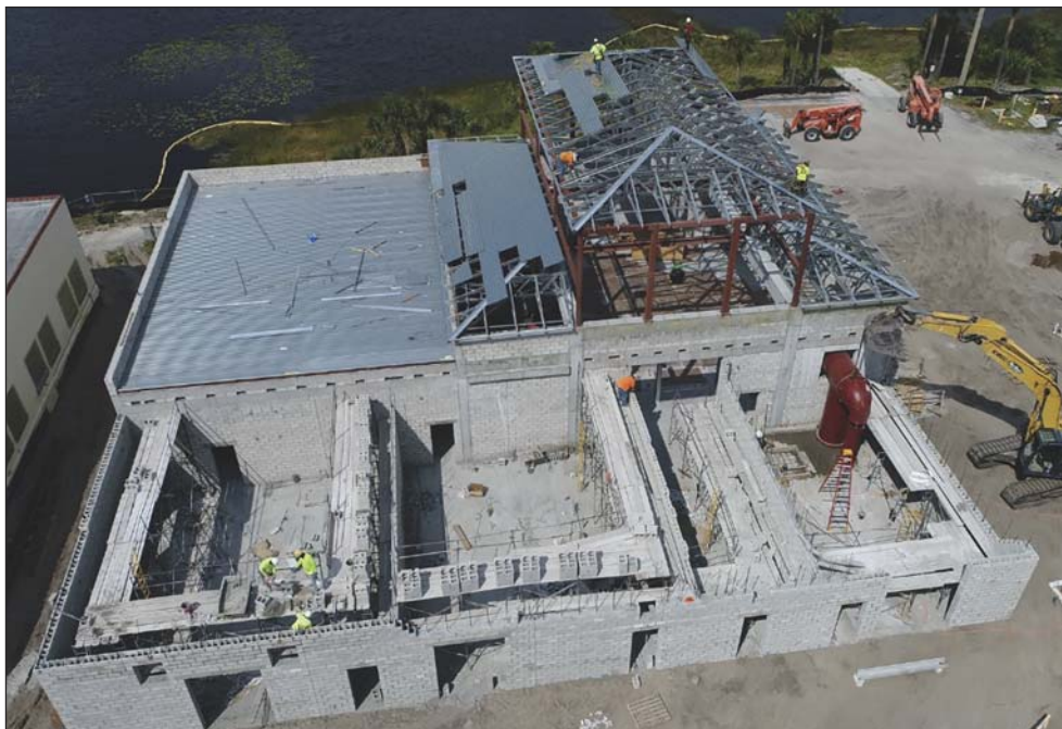
Figure 9. Transfer/Ultraviolet Building Construction (photo: Stantec)
