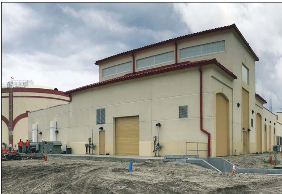
Figure 11. Transfer/Ultraviolet Building Nearing Completion (photo: Stantec)
