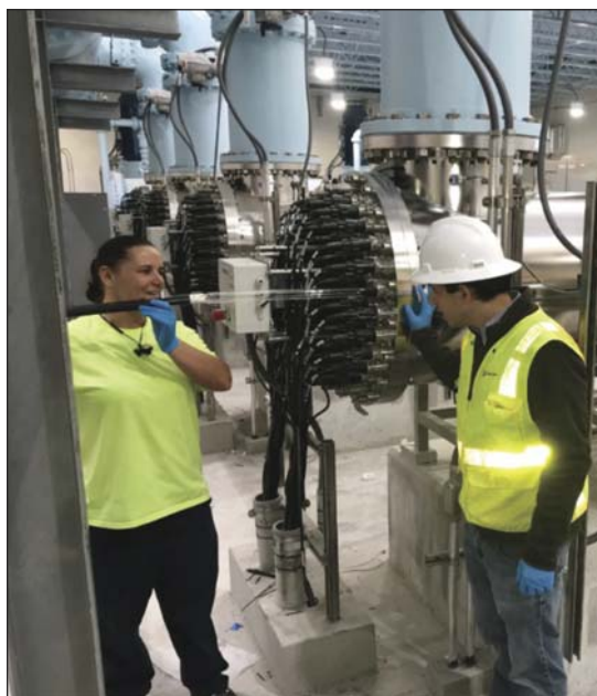
Figure 10. Ultraviolet Bulb Replacement Training (photo: Stantec)
