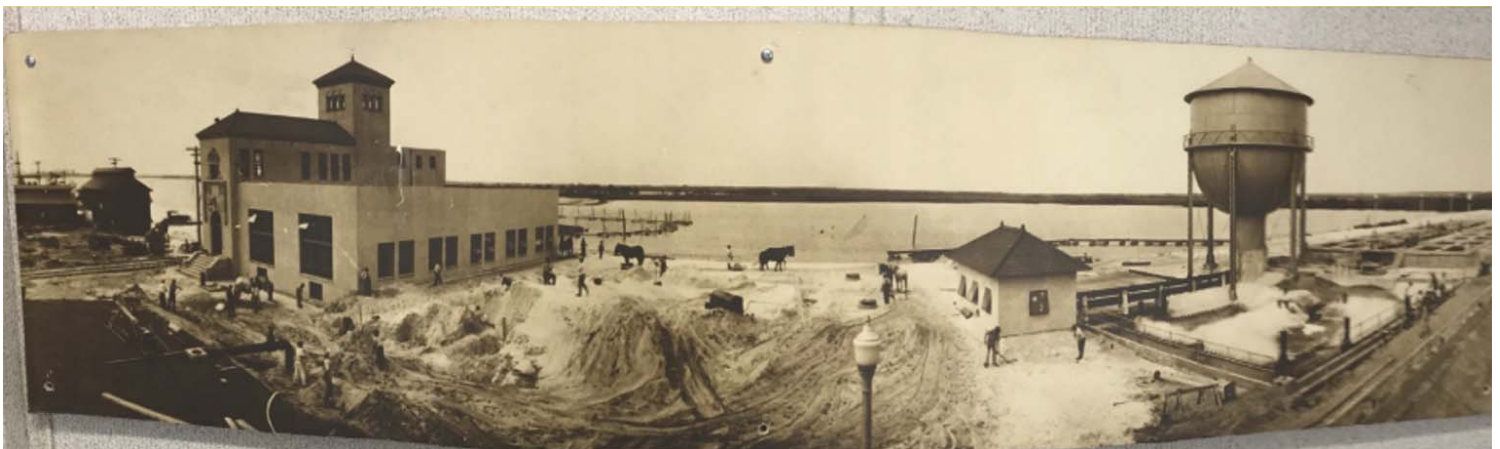
Figure 1. 1926 Pump Station Panoramic (photo: City of West Palm Beach)
