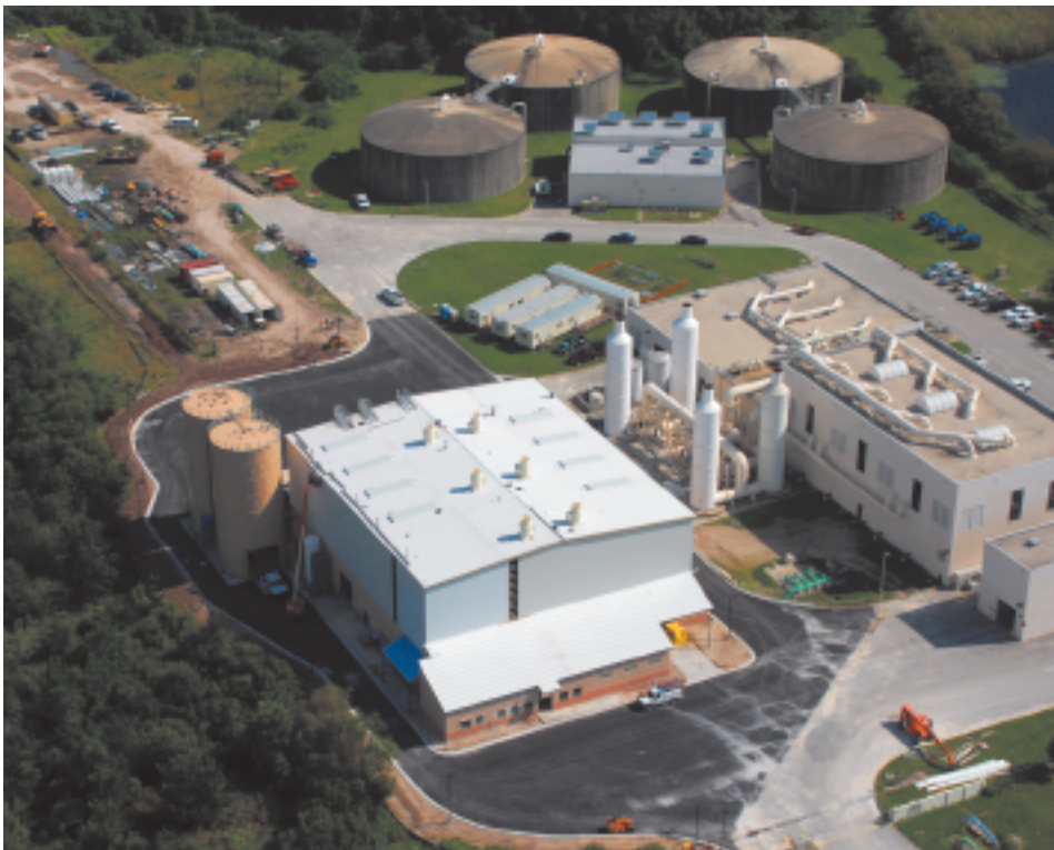
The Hillsborough County Biosolids Management Facility.
