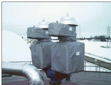
Figure 9. Pressure-reducing valve (PRV)/flame arrester with insulating jacket.
