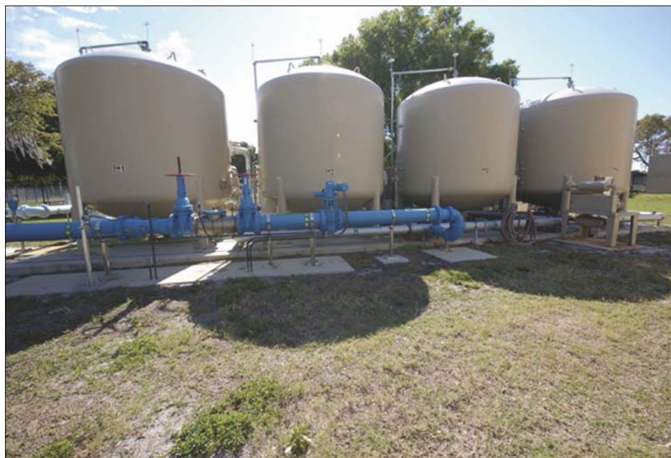
Pressure filters considered for preliminary design.
