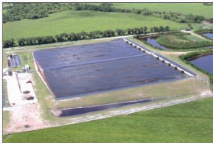
Figure 6 – HydroMentia ATS S-154 Basin Facility in Okeechobee County, FL (Stewart, E.A. 2007)
