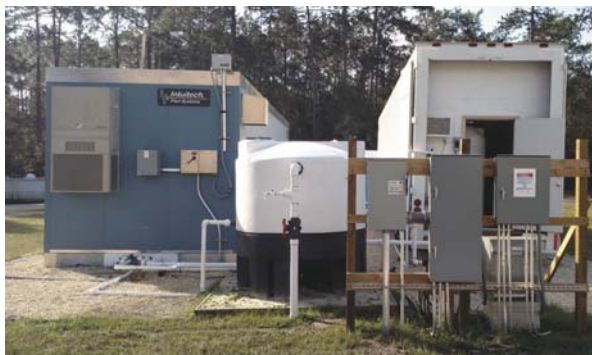
Figure 2. Ultrafiltration/Reverse Osmosis Process
