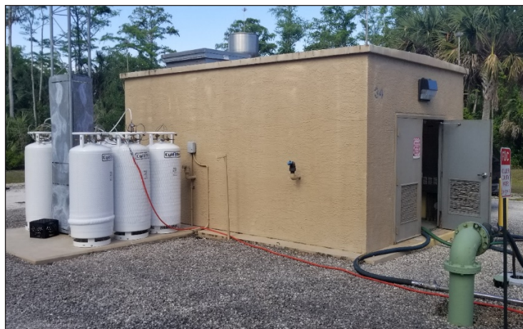
Figure 4. Carbon dioxide injection tanks and raw water main connection.
