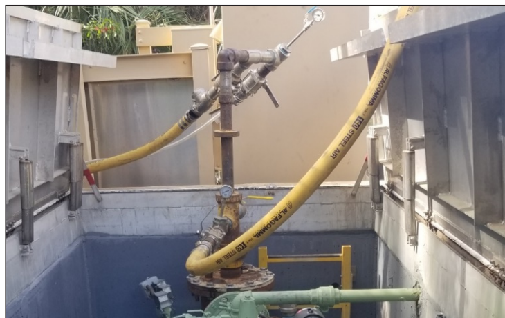
Figure 5. Acid header assembly at wellhead.
