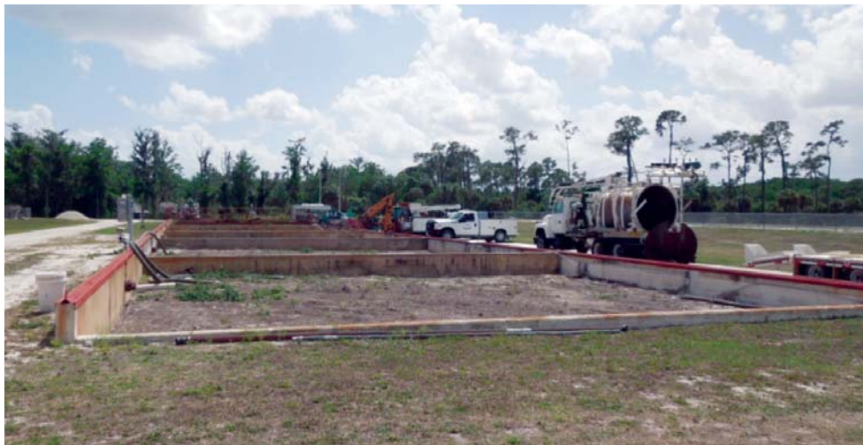
Figure 8. Project Area Before Construction
