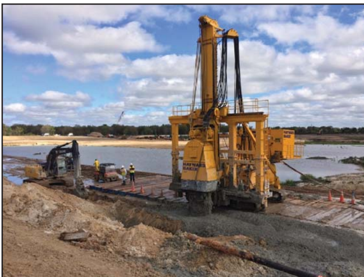
Figure 3. Trench Remixing and Cutting Deep Wall (TRD) Installation
