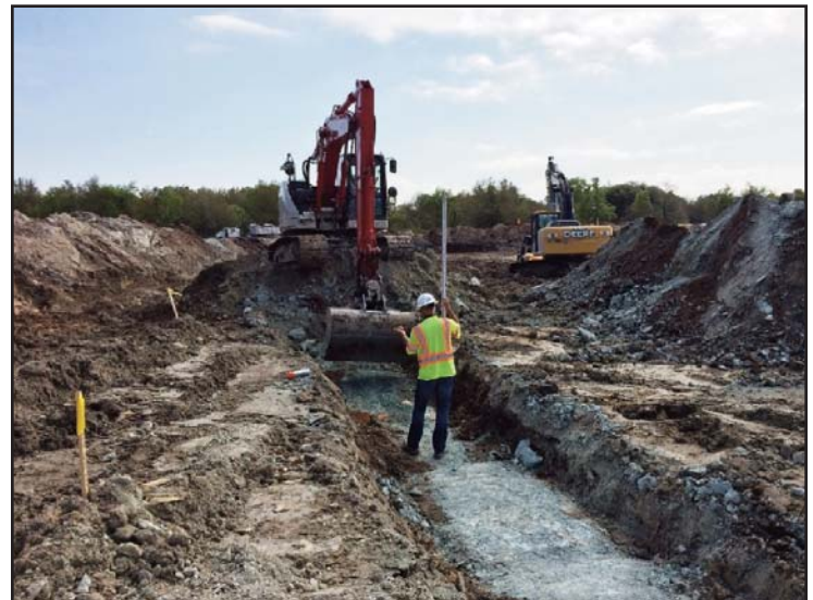
Figure 4. Trench Remixing and Cutting Deep Wall (TRD) Completed On-Site
