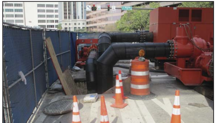
Figure 11. Installed Bypass System Components: Average-Flow Pumps and Enclosure
