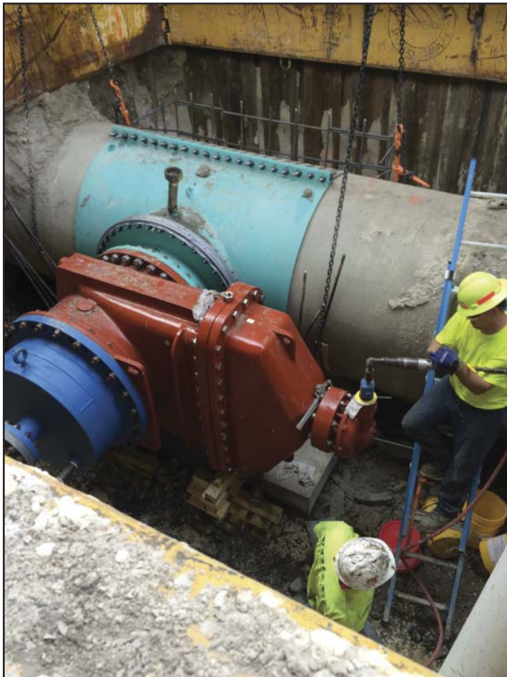
Figure 10. 54-in. x 36-in. Hot Tap on Prestressed Concrete Cylinder Pipe
