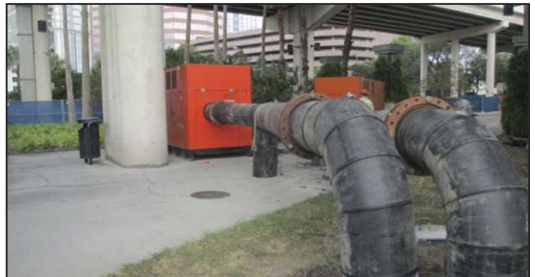
Figure 12. Installed Bypass System Components: Peak-Flow Pumps
