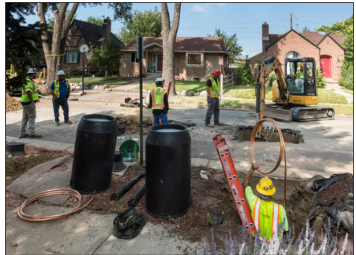
Lead service line replacement plans are due by October 2024. Though replacement may not be required, the availability of funding should make lead service line replacement a priority.
