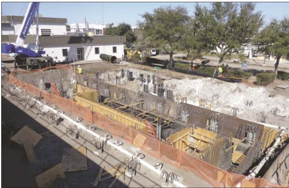
Figure 6. Piping and Encasement Installation Below the Biological Treatment Unit
