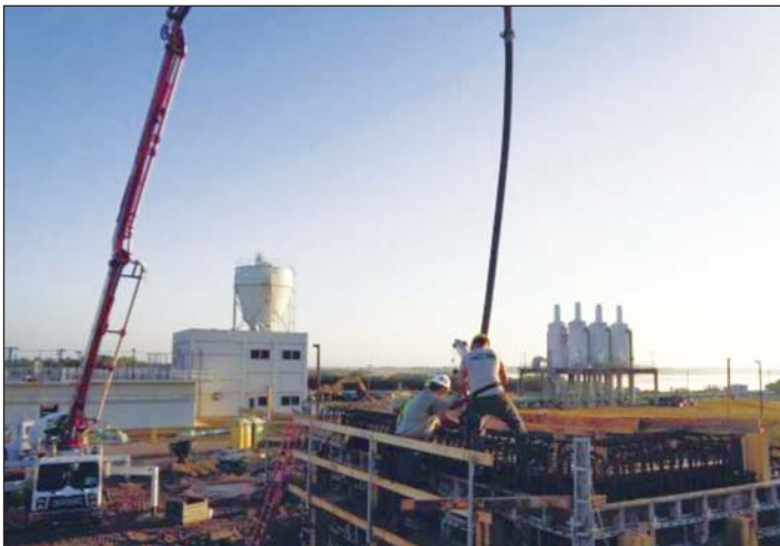
Figure 7. Concrete Pour for the Backwash Pump Station
