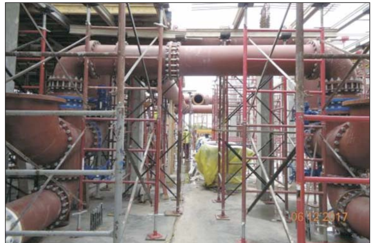
Figure 8. Pipe Gallery and Second-Floor Elevated Slab Construction
