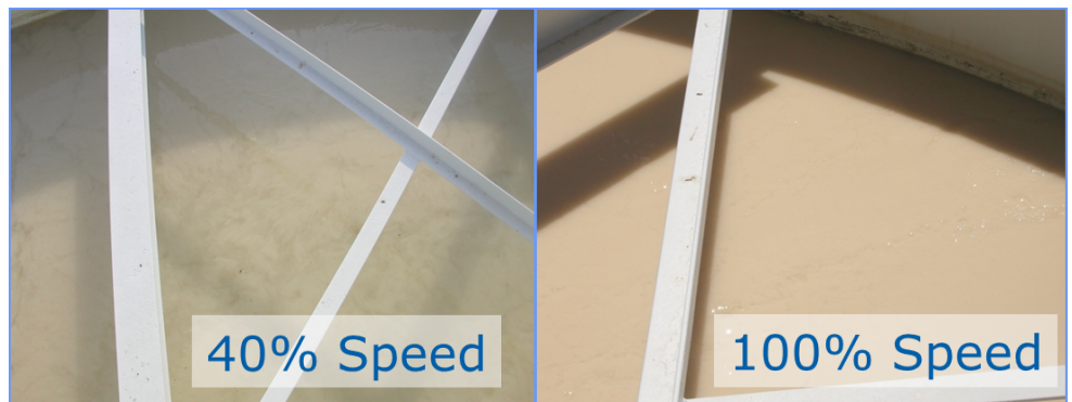
Figure 4. Center Cone Solids at Varying Mixer Speeds (Recirculation Ratios)
