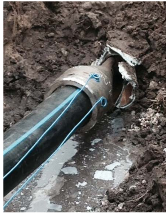
Photo 2. Asbestos Cement Pipe Bursting
