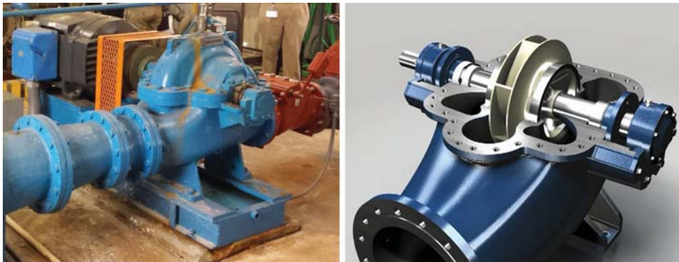
Figure 1. Horizontal split case pump in a pump station building (left) and the same kind of pump with the top case removed (right).
