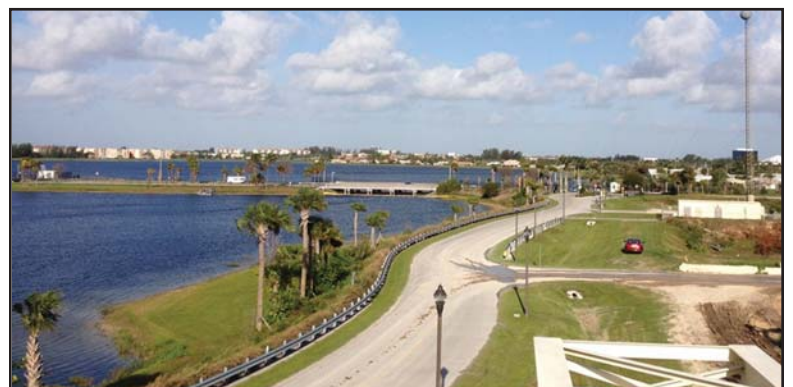
Figure 3. Safe Access Driveway from Australian Avenue.
