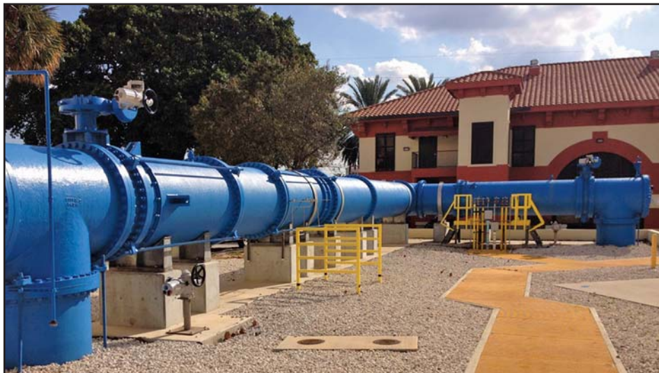
Figure 6. Mixing and Metering Header.
