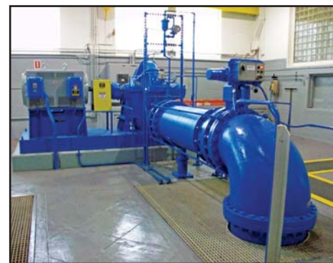
Figure 9. High-Service Pump No. 7.
