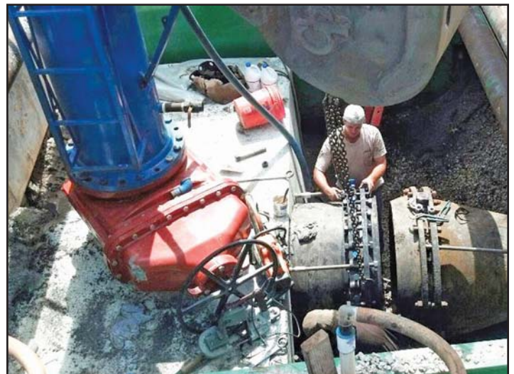
Figure 5. 42-in. Line Stop to Bypass In-Service Water Main Supplying.
