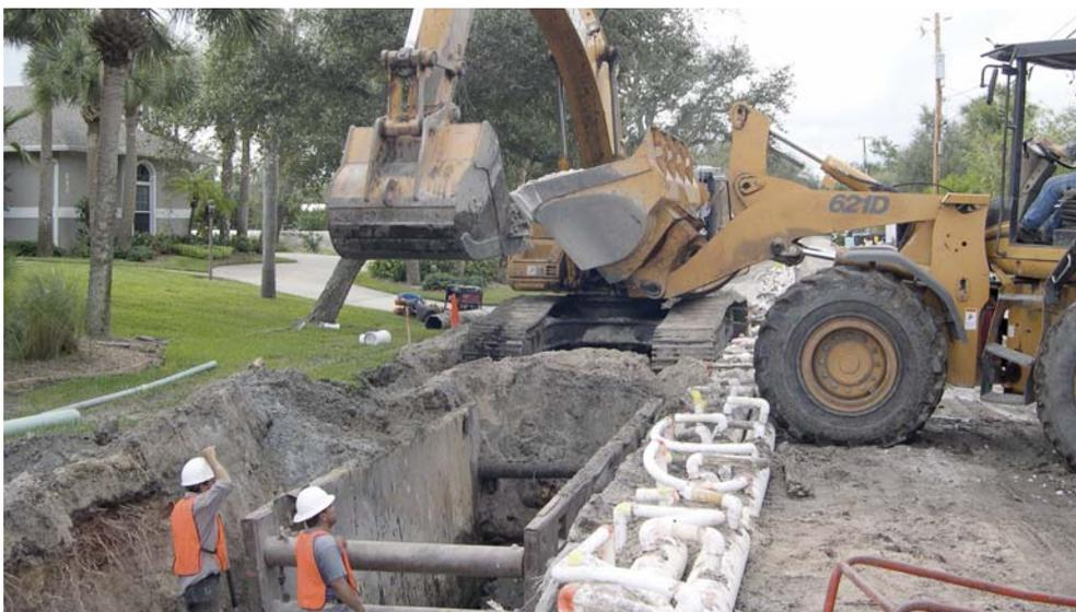
Figure 4. Gravity sewer main excavation.
