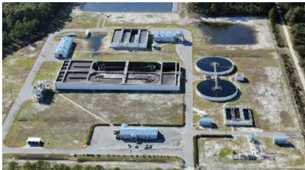
Military Point Regional Advanced Wastewater Treatment Facility
