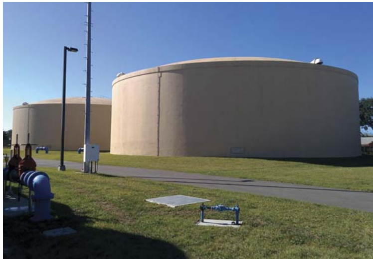
The new ground storage tanks.
