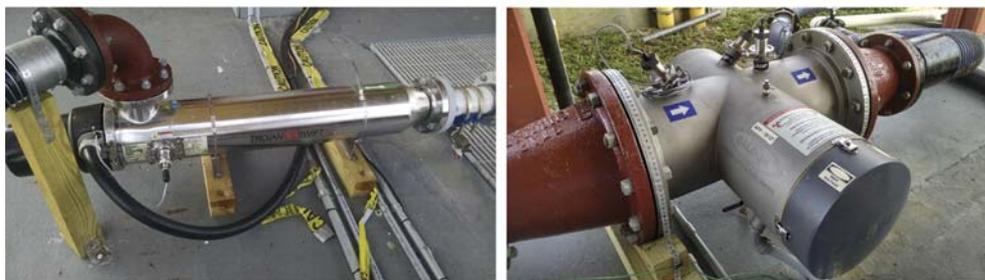
(a) Low-Pressure High-Output and (b) Medium-Pressure
