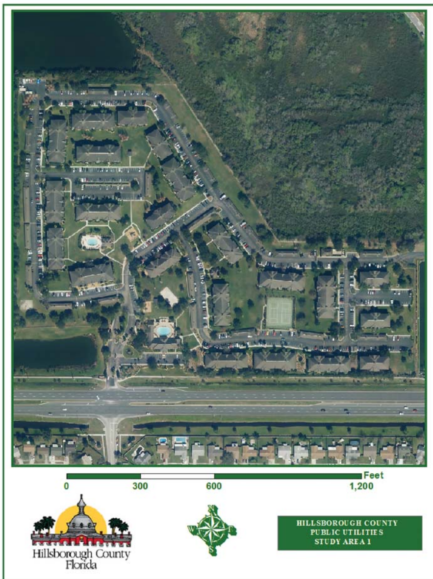
Figure 1. Aerial View of Study Area 1
